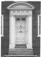
③ A decrease of c. 1740-50 in which the arched top of the door void breaks into the pediment, etc.
