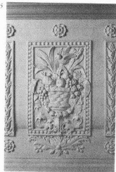
⑤ A plaster dado infill panel. It is unusual to find this degree of elaborate detail in Edwardian plasterwork. EL
