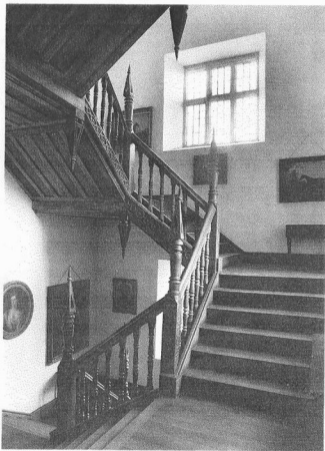
This is the principal staircase at Chastleton House, Oxfordshire, 1602. It is of the framed type (without a central newel). The
