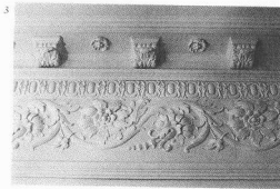
⑤ A plaster dado infill panel. It is unusual to find this degree of elaborate detail in Edwardian plasterwork. EL
