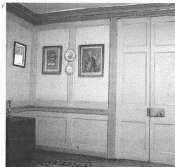
① The dividing wall between front and back rooms in a typical 1720s town house. The tall doors are detailed en suite with the other panelling. DC
