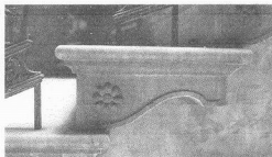
② In grand houses, the handrail on main stairs was finely moulded and terminated in a spiral, be it a tight coil or, as here, a loose curve. 181
