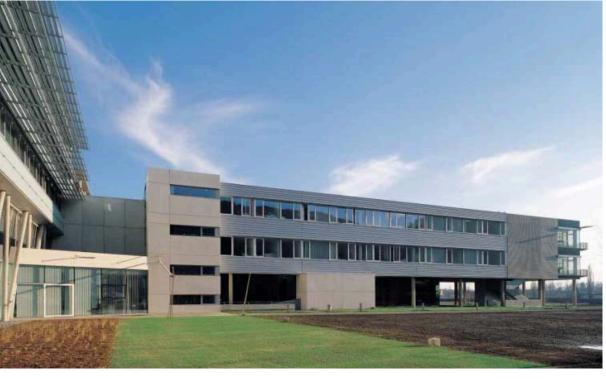
In a nod to nature's healing powers, the architects placed patient rooms along the perimeters of each wing (top); some even have balconies (bottom). Brushed metallic louvers (at right in bottom photo) prevent excess heat gain and minimize the need for air-conditioning.
