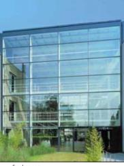
Technical Glass Products offers the Fireframes™ Curtainwall Seriesfire-rated steel framing for large expanses of glass spanning multiple stories. Available for interior or exterior use, the Curtainwall Series carries fire ratings up to two hours. Custom exterior face caps allow a wide variety of appearances, including stainless steel. For more information visit the company's Web site.
