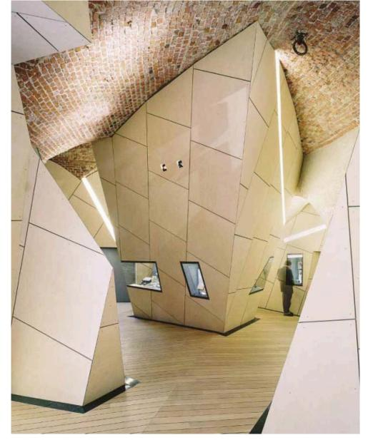
Glazed vitrines project forward from freestanding objects (below), including ones shaped like the hull of a boat (left). The sloping oak-plank floor seems to float between the ventilation scuppers (opposite) and is carried by joists over a concrete slab.
