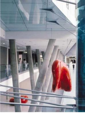
Partitions in the reception area, including the elevator shafts, are made of glass, whether clear, tinted, or frosted. Even the ends of the corridors parallel to the long axes of each wing are glazed, so that neither patients nor staff ever lose sight of the bucolic outdoors. The architects used metallic louvers outside and oriented the building to minimize the need for air-conditioning. Natural cross ventilation in the patient wings adds to the delight of abundant natural lighting.
