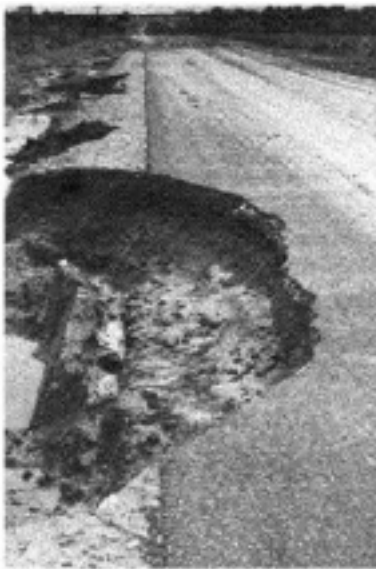
Figure 4-1. Roadway Base Failure
