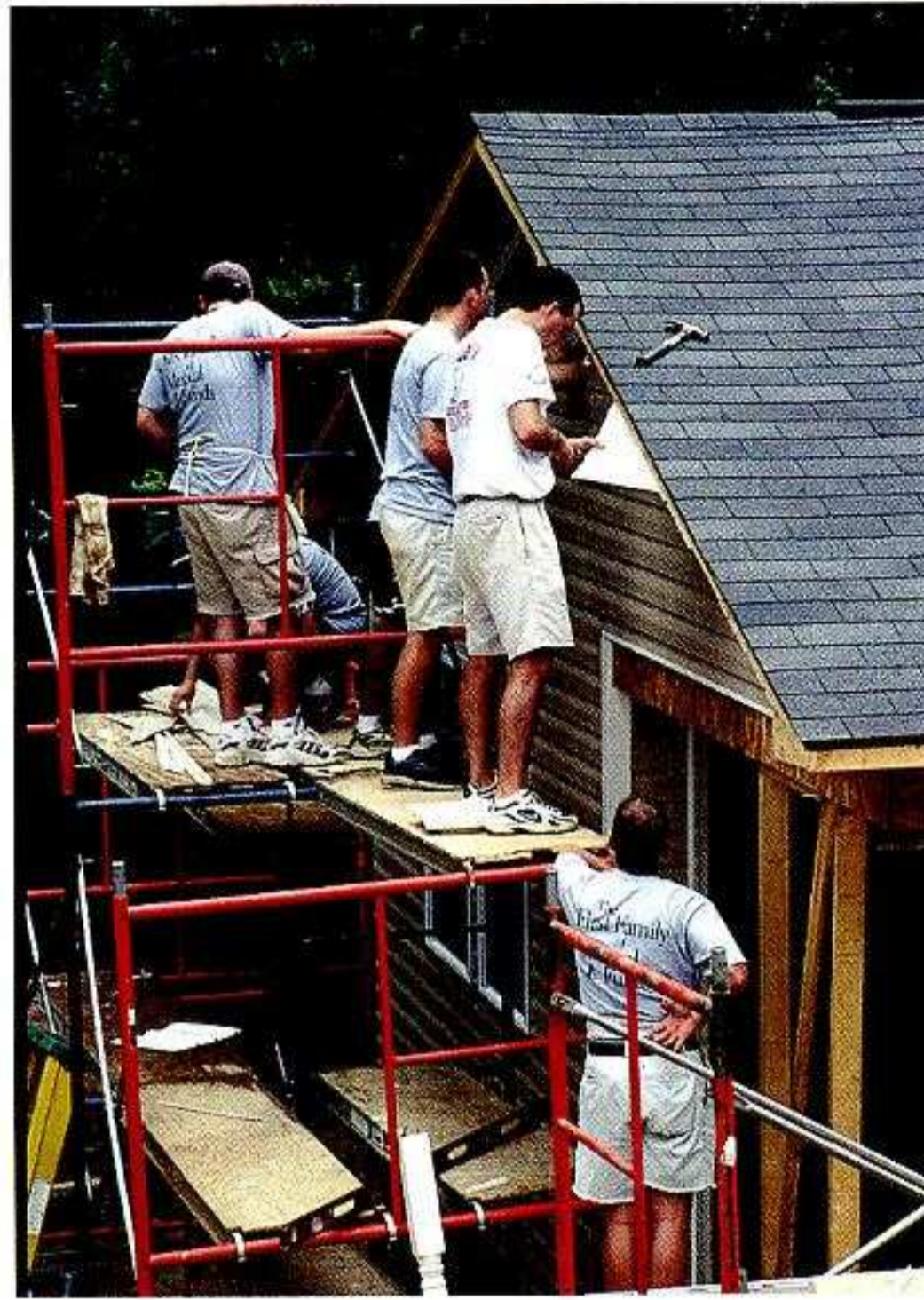
FINISHING VINYL-SIDING WORK
