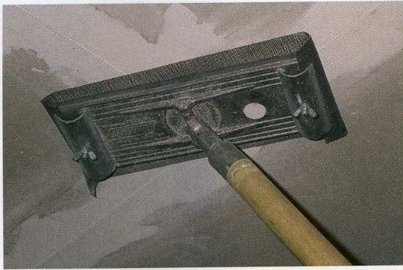
SMOOTH THE JOINT COMPOUND. A sanding screen attached to the plate on the end of a sanding pole allows you to smooth joint compound rapidly. [Photo © The Taunton Press, Inc.]
