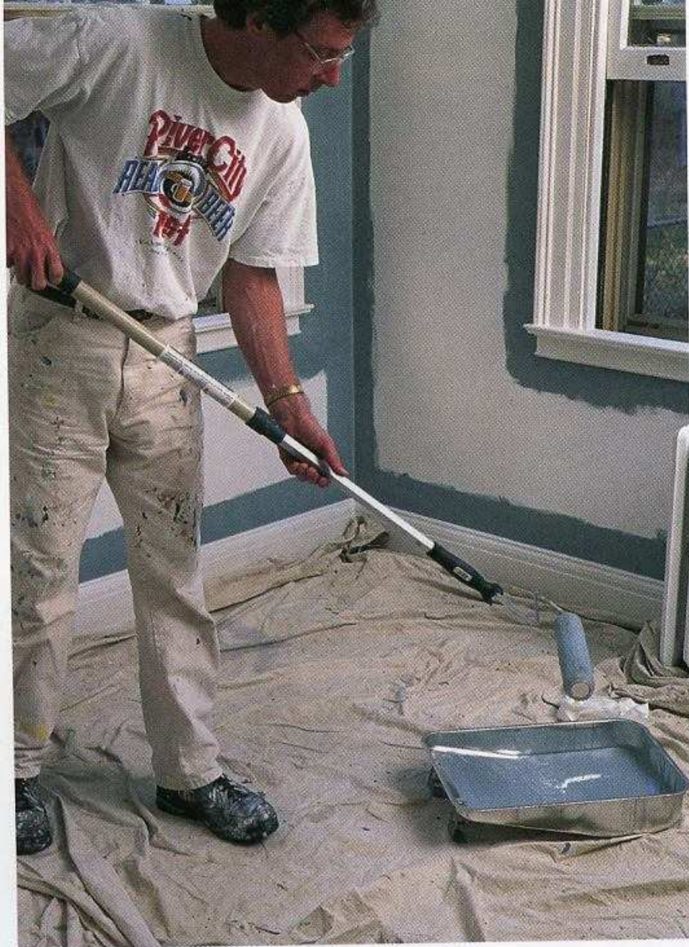
LOAD YOUR ROLLER IN A RIBBED PAN. To control the amount of paint in a roller and minimize spills and splatters, work the roller back and forth along the upper ribbed part of the pan. [Photo © The Taunton Press, Inc.]
