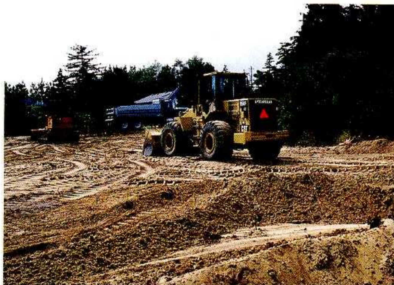
PREPARING THE SITE
