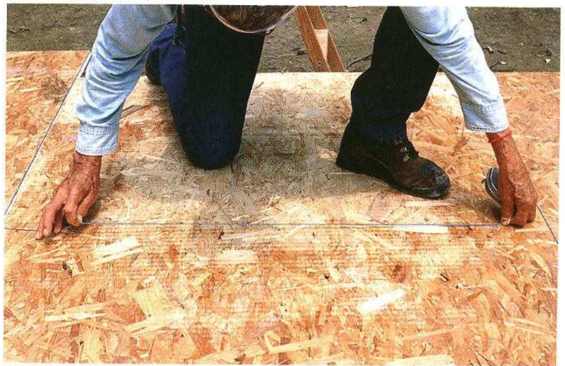
SNAP A LINE. Loaded with powdered chalk, a chalkline stretched tightly between two points is snapped to make straight lines quickly and accurately.
