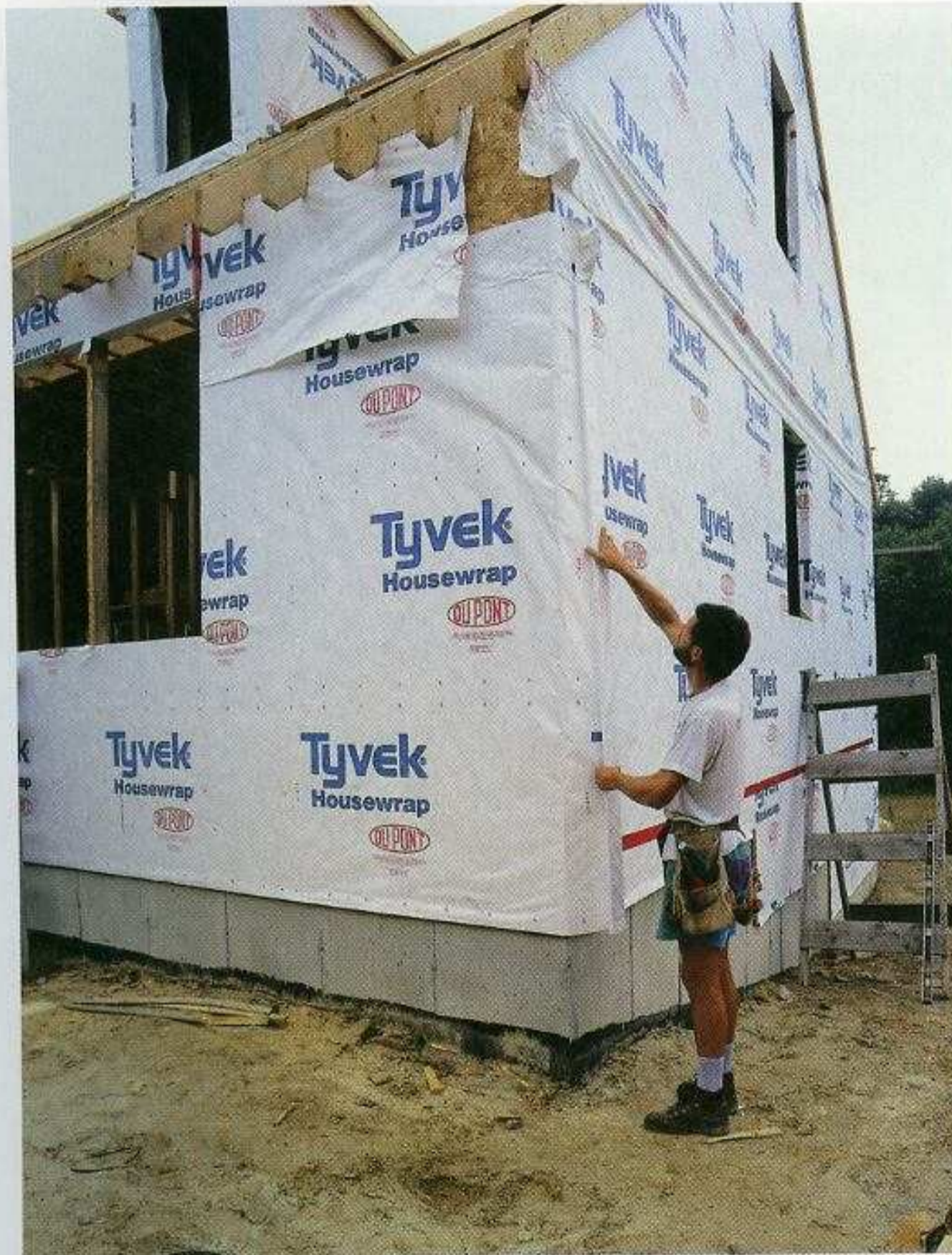
HOUSEWRAP ACTS AS A WATERPROOF WINDBREAKER. Tyvek and other modern housewraps are installed beneath the exterior siding. They block wind and water while still allowing vapor to pass through. [Photo © Mike Guertin.]
