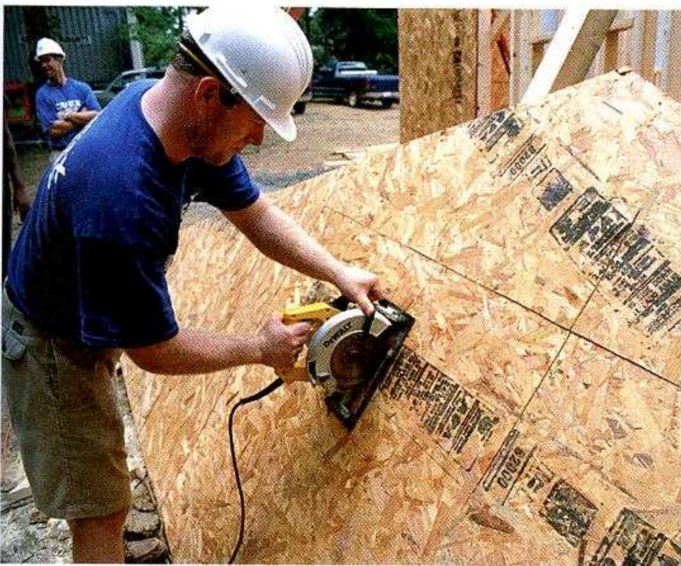
DIRECT-DRIVE SAW. Sometimes referred to as a sidewinder saw, a direct-drive saw is a type of circular saw. Its motor is on the side, in line with the blade.
