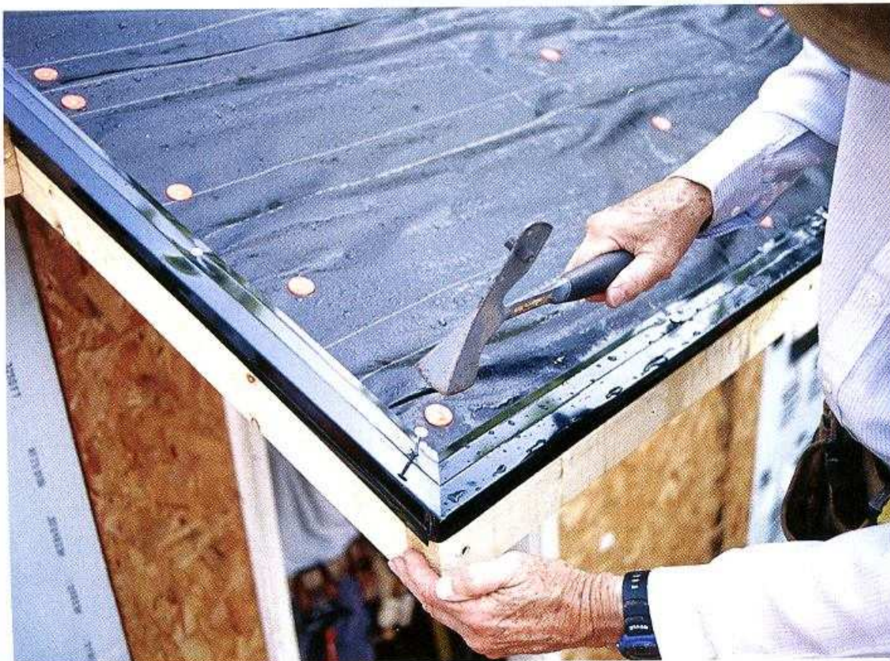
INSTALLING A DRIP EDGE. This L-profile flashing is installed around the edges of the roof.
