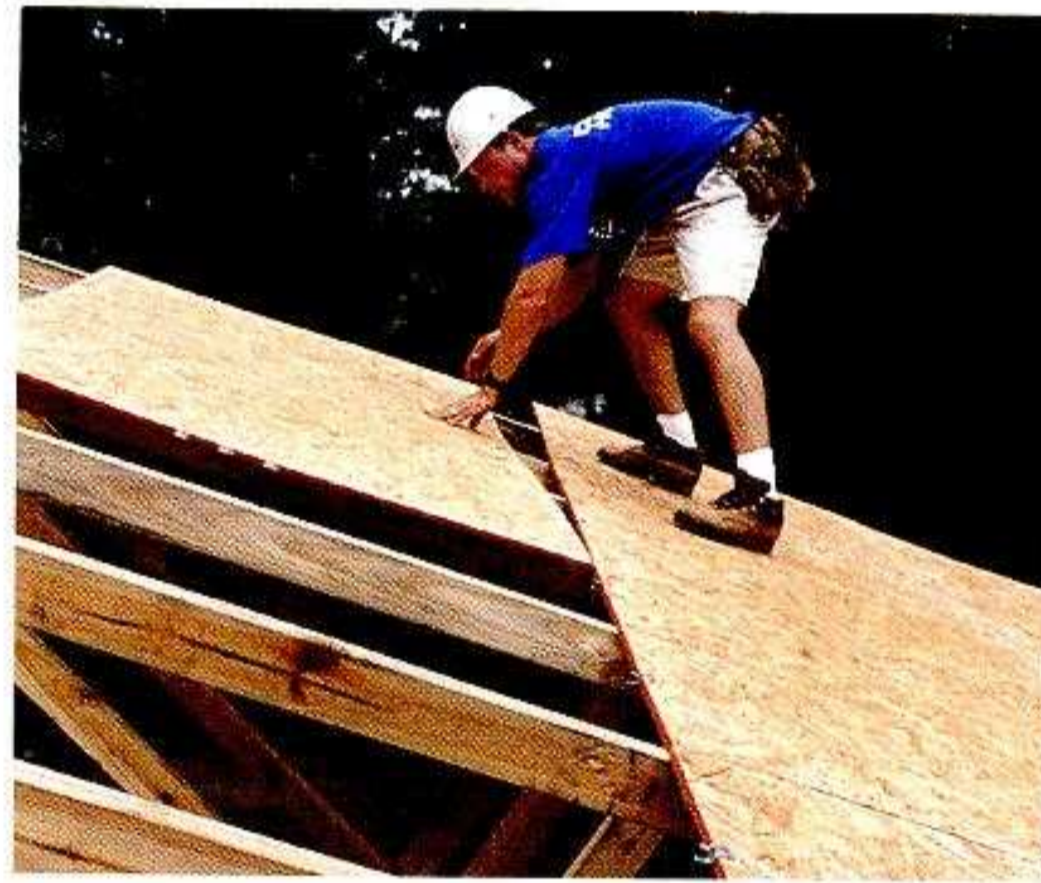
SHEATHING THE ROOF
