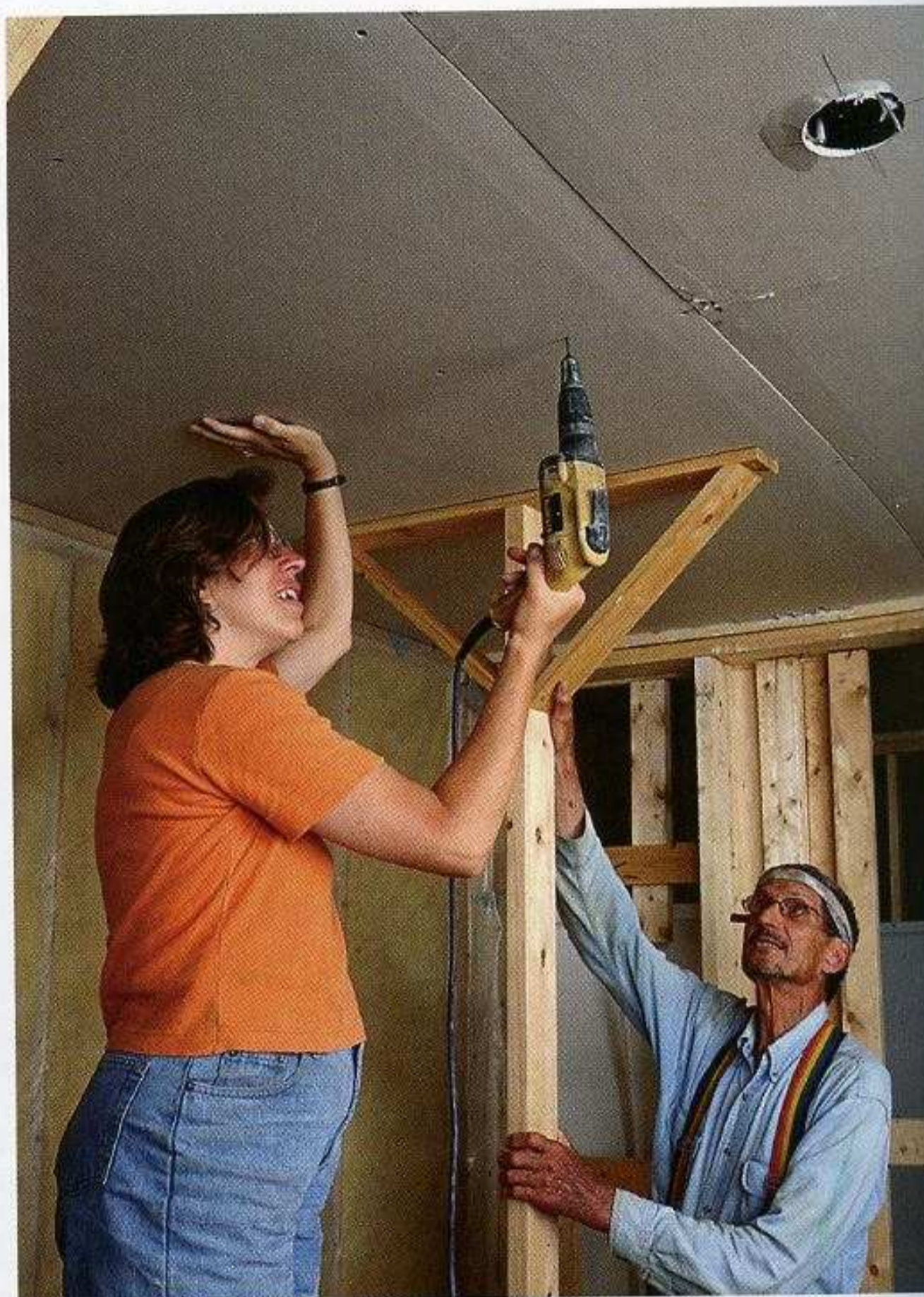
USE A SCREW GUN. This electric drill is designed to drive drywall screws to exactly the right depth.
