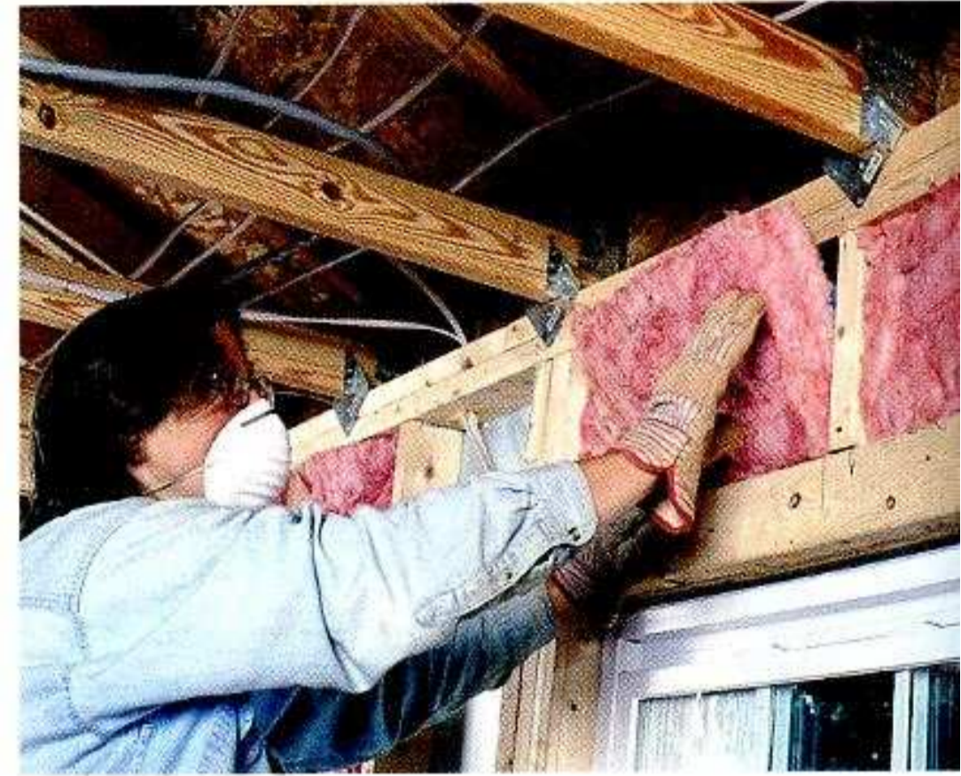
INSTALLING FIBERGLASS BATT INSULATION
