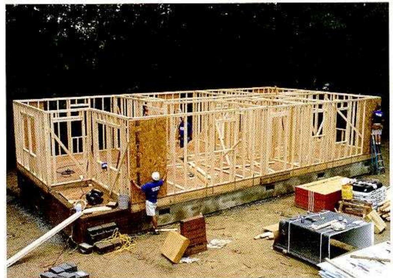
BEGINNING TO SHEATHE THE WALLS
