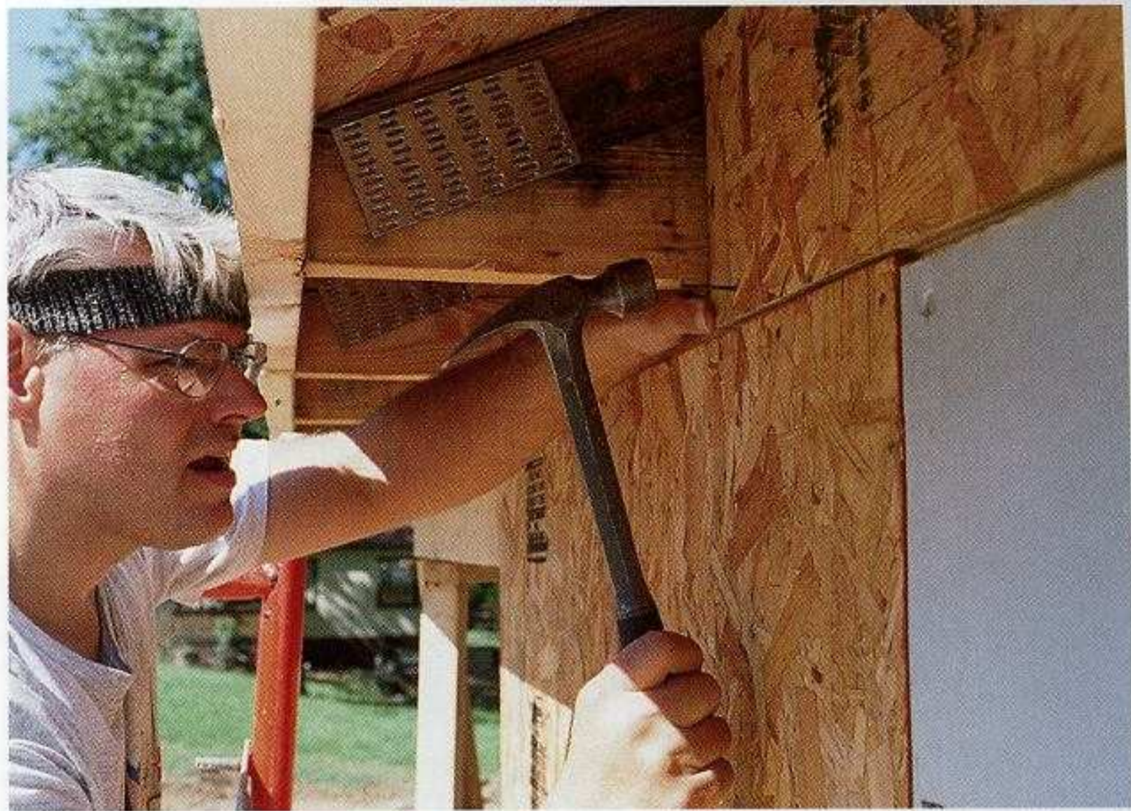
BAFFLES KEEP INSULATION OUT OF THE EAVES. Nail these panels to the top of the wall between the roof trusses.
