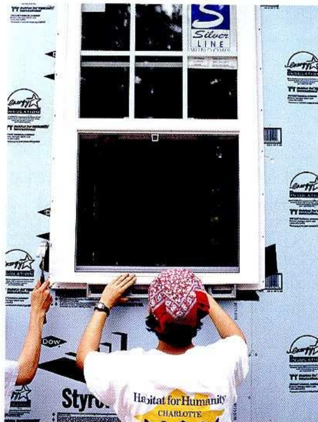
INSTALLING A WINDOW
