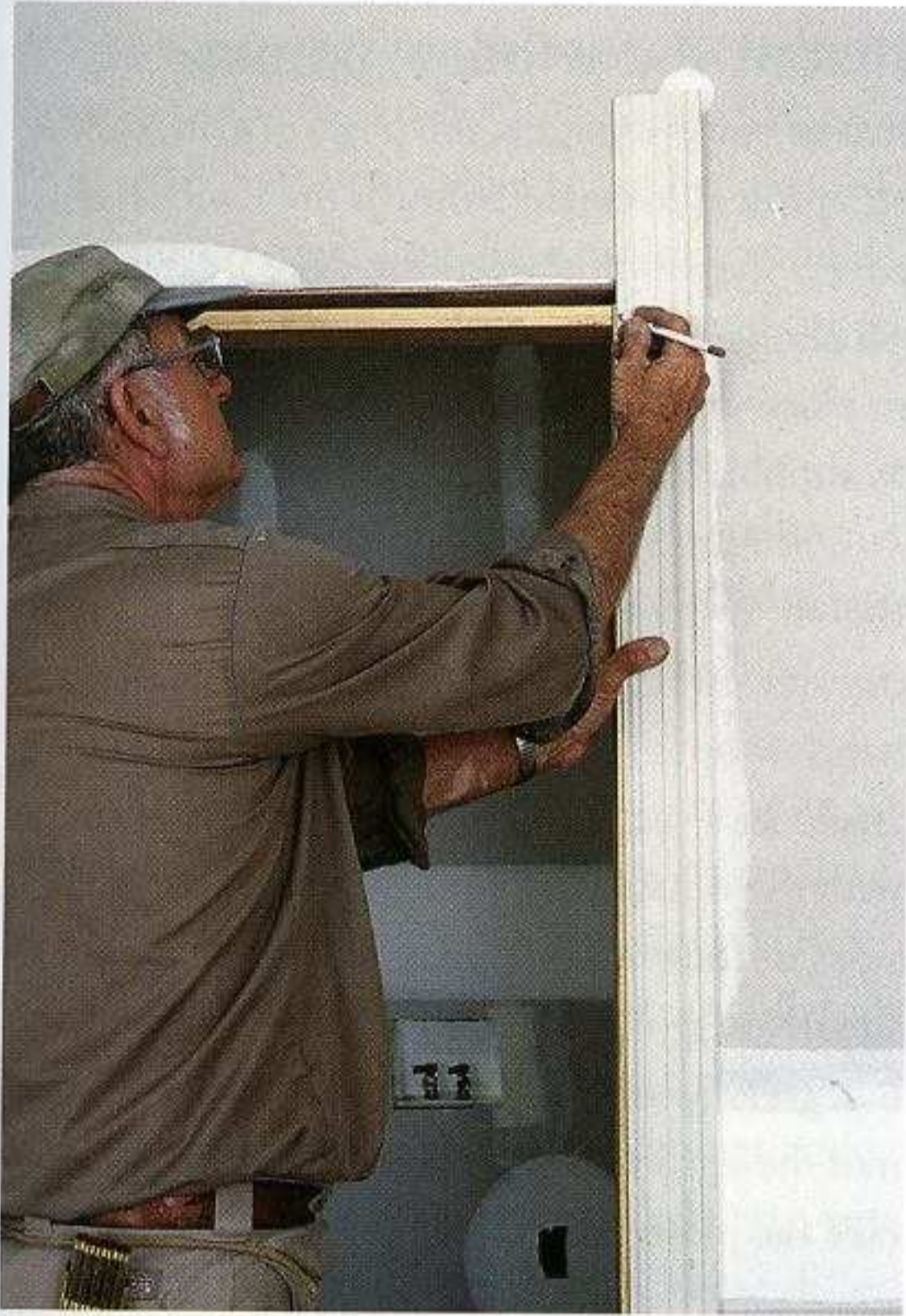
MARK THE CASING; DON'T MEASURE. Mark the short end of the casing's miter cut by holding the casing in place on the jamb.
