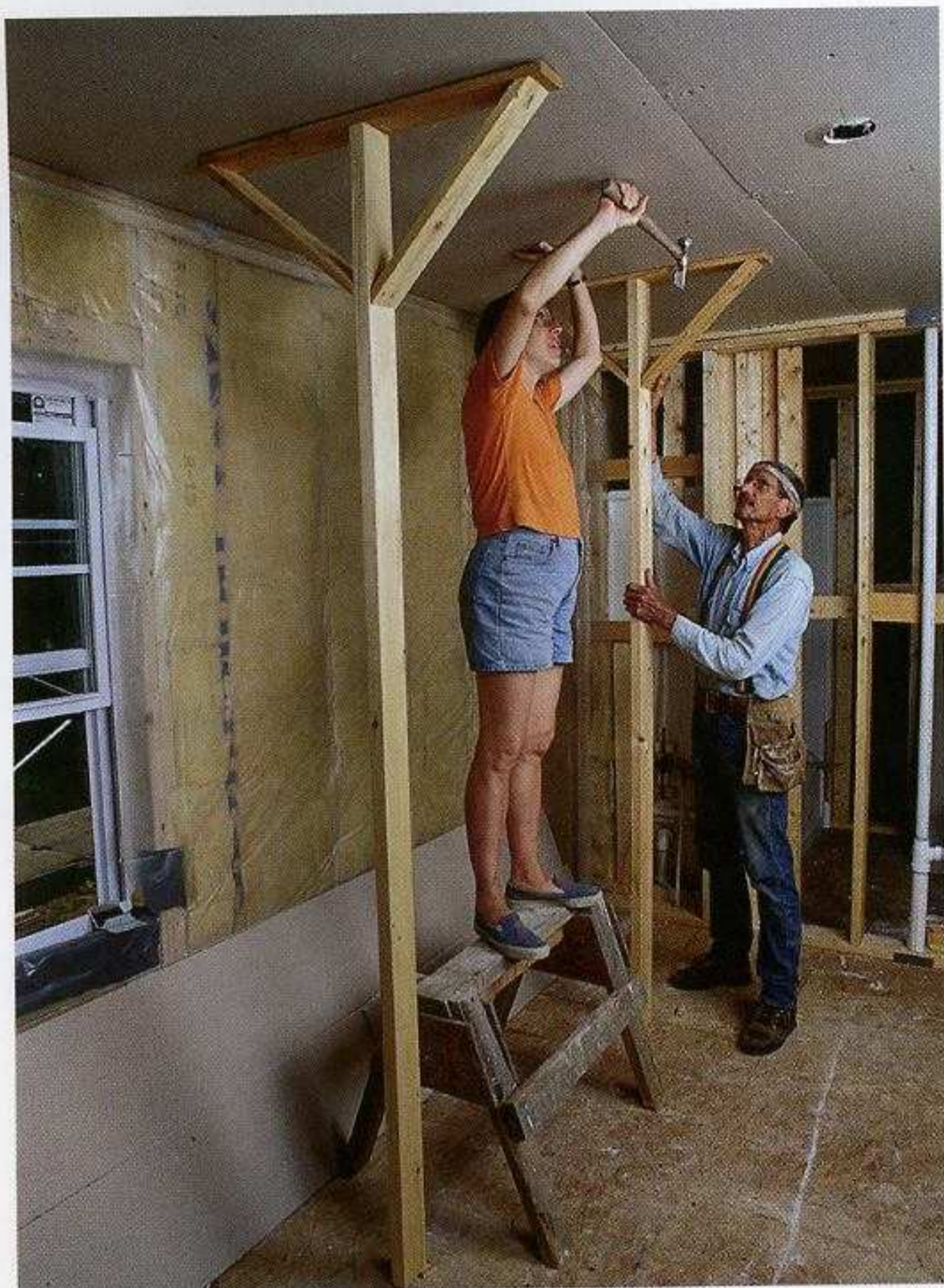
T-SUPPORTS ARE HELPFUL HOLDERS. Easily made on the job site, T-supports hold ceiling panels in place, allowing you to concentrate on driving nails or screws.
