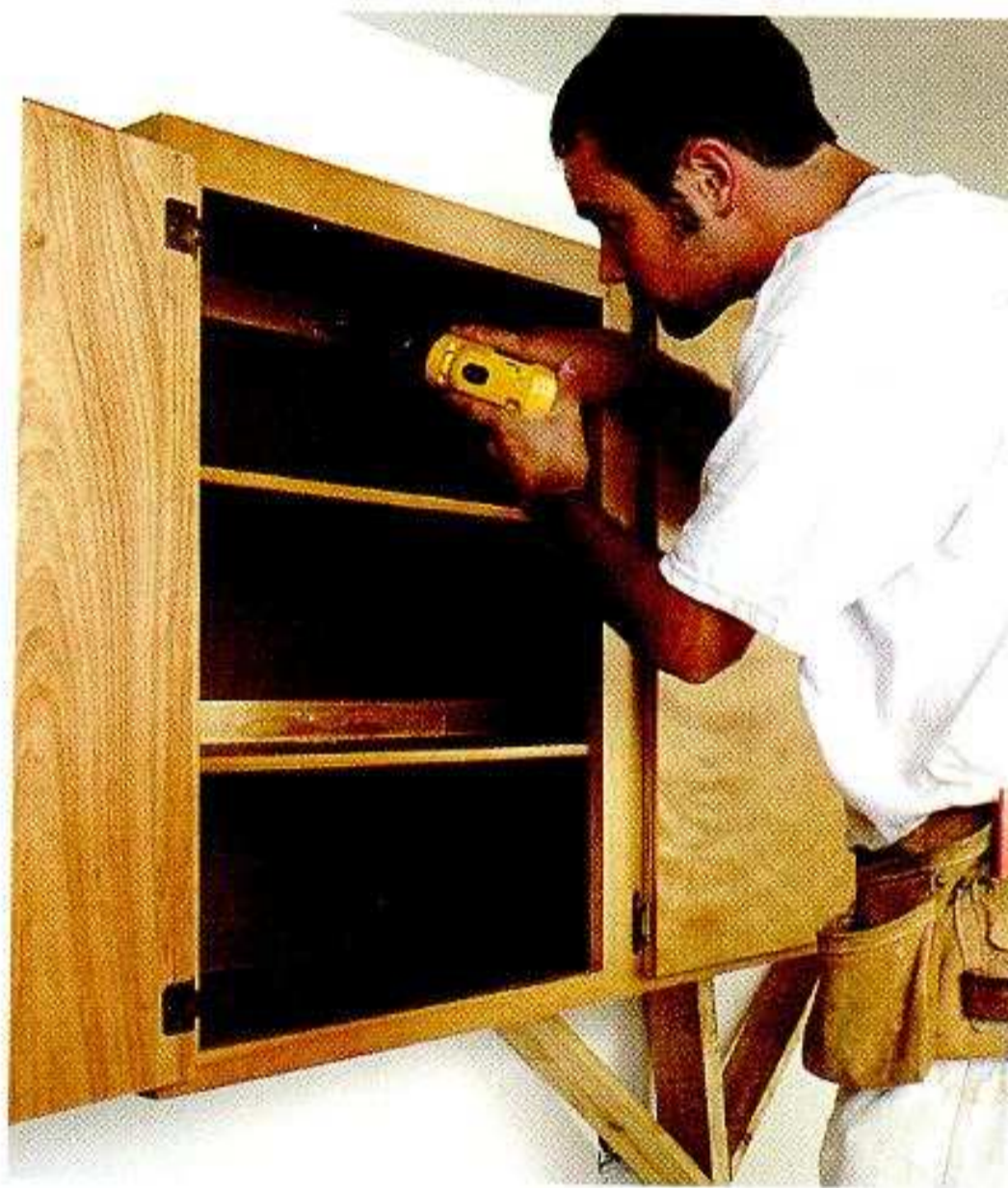
INSTALLING A WALL CABINET
