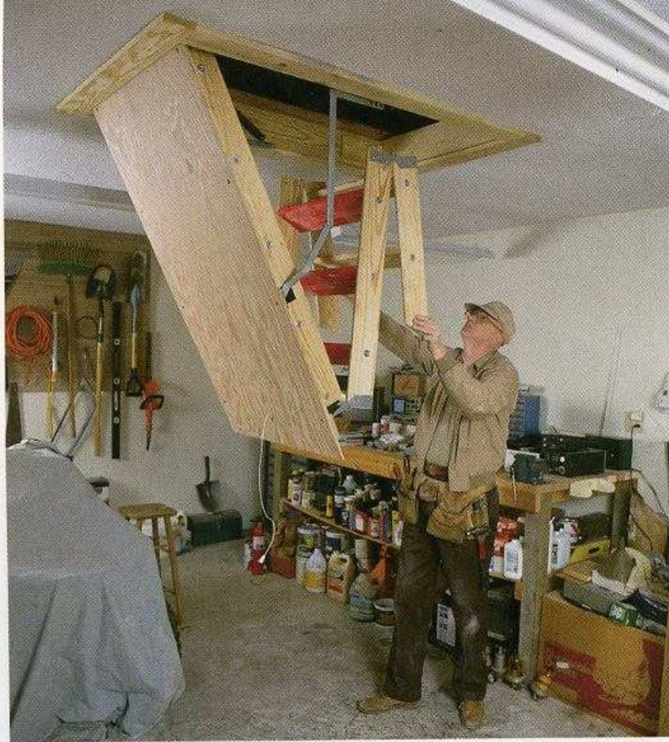
A DROP-DOWN STAIRCASE PROVIDES EASY ACCESS. Installing a factory-made folding staircase lets you gain convenient access to attic space. [Photo by Jefferson Kolle, courtesy Fine Homebuilding magazine, © The Taunton Press, Inc.]
