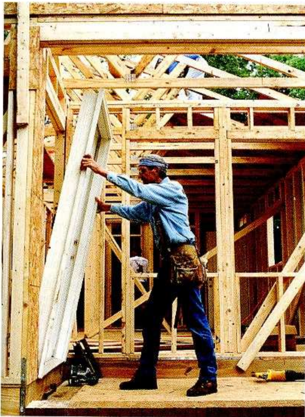
TEST-FITTING THE FRONT DOOR
