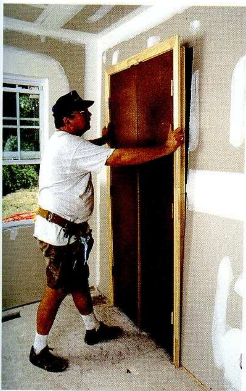
INSTALLING AN INTERIOR PREHUNG DOOR
