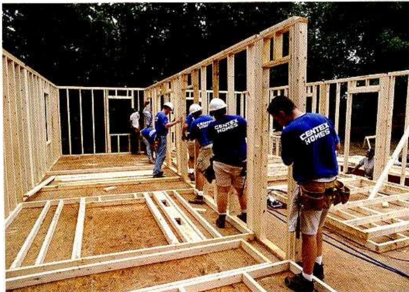
RAISING THE WALLS
