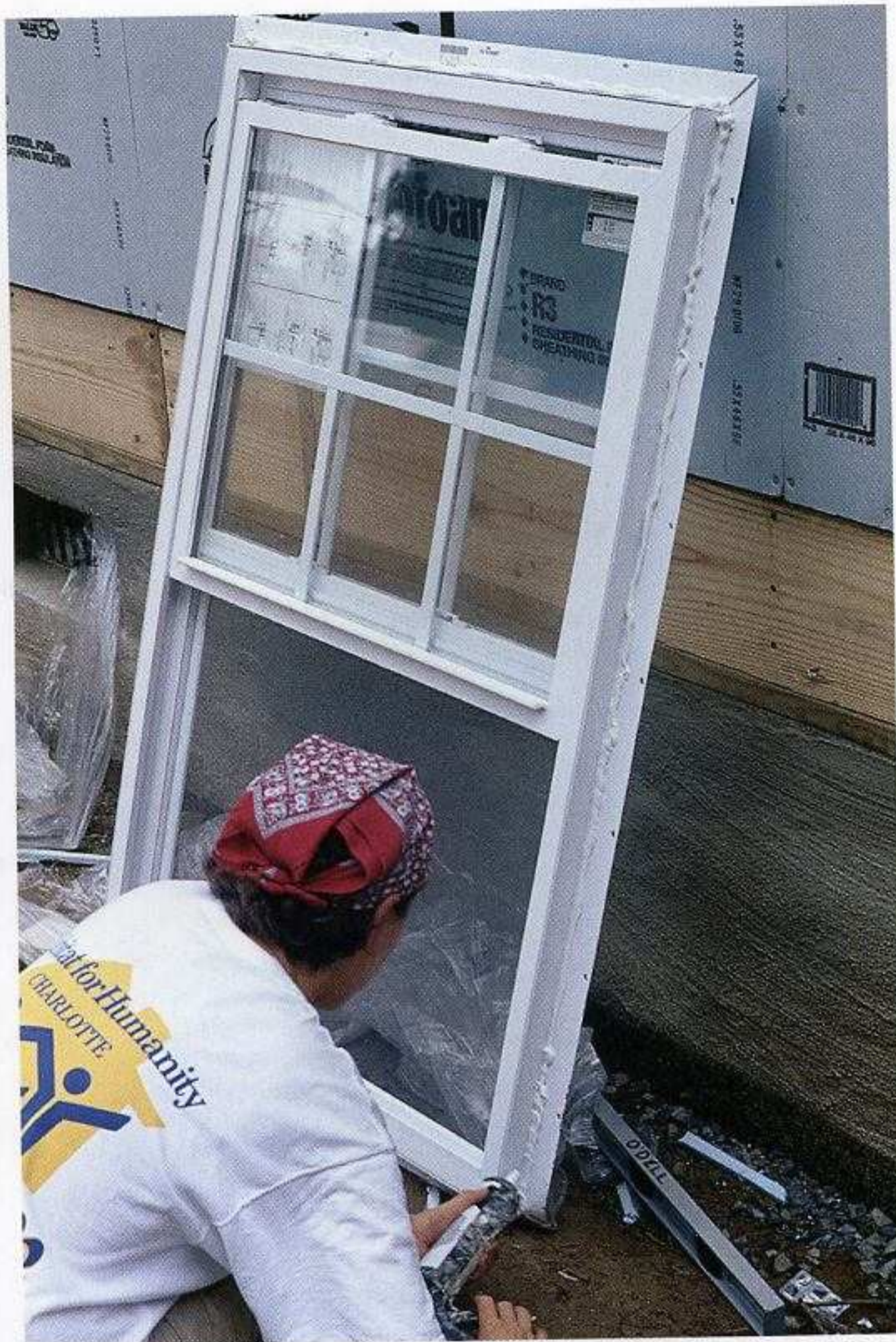
FLANGED WINDOWS ARE EASY TO INSTALL. Before setting the window in its opening, apply exterior caulk to the flange surface.
