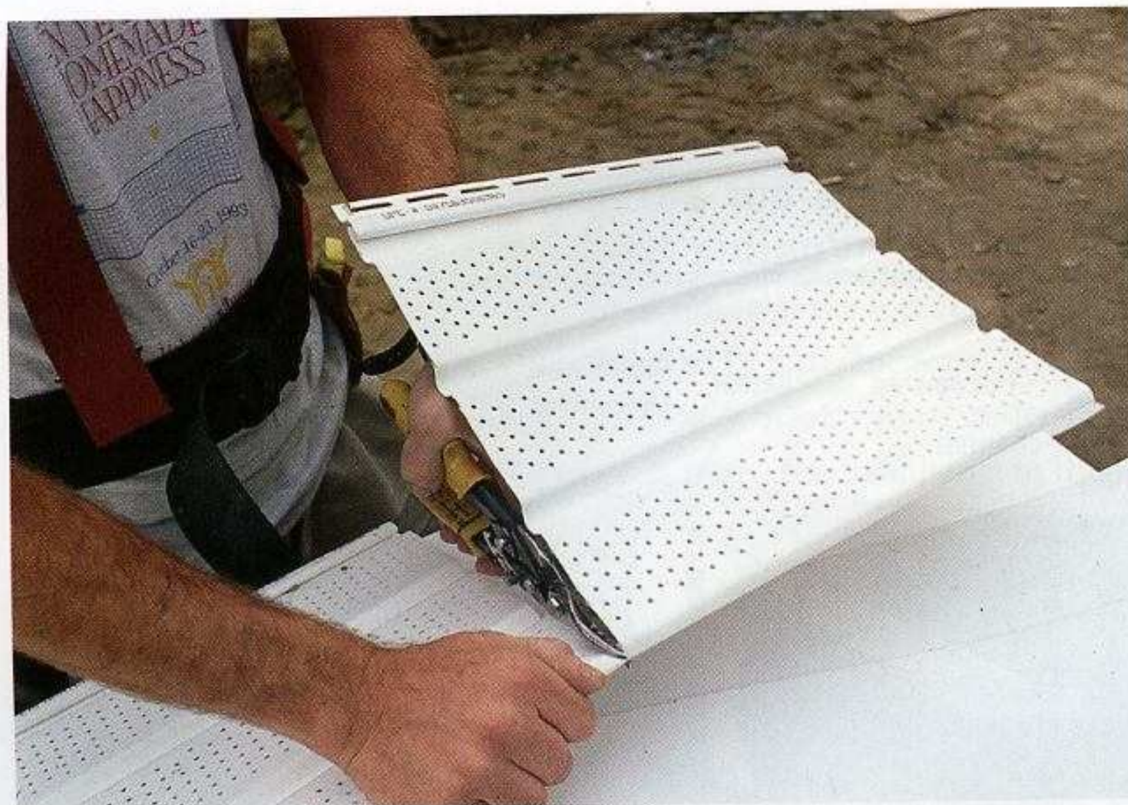
CUT SOFFIT PANELING. Perforations in vinyl soffit material allow ventilation through the eaves. The soffit panel has a nailing flange with slotted holes similar to those found on vinyl siding. Cut panels to size with metal shears.
