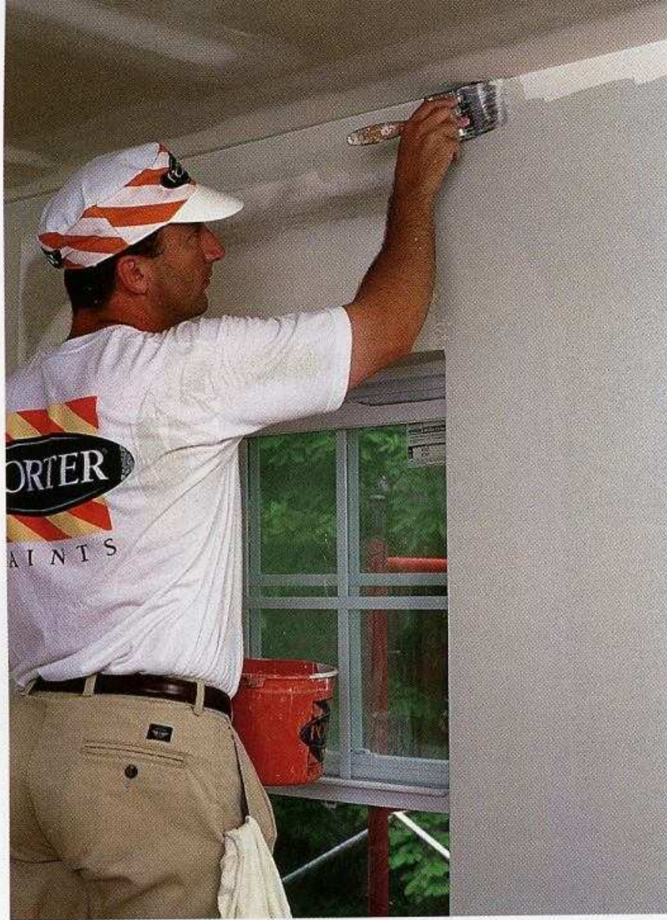
CUT IN WITH A PAINT BRUSH. A roller can't reach corners and edges. A 3-in.- to 4-in.-wide brush is ideal for painting these areas.
