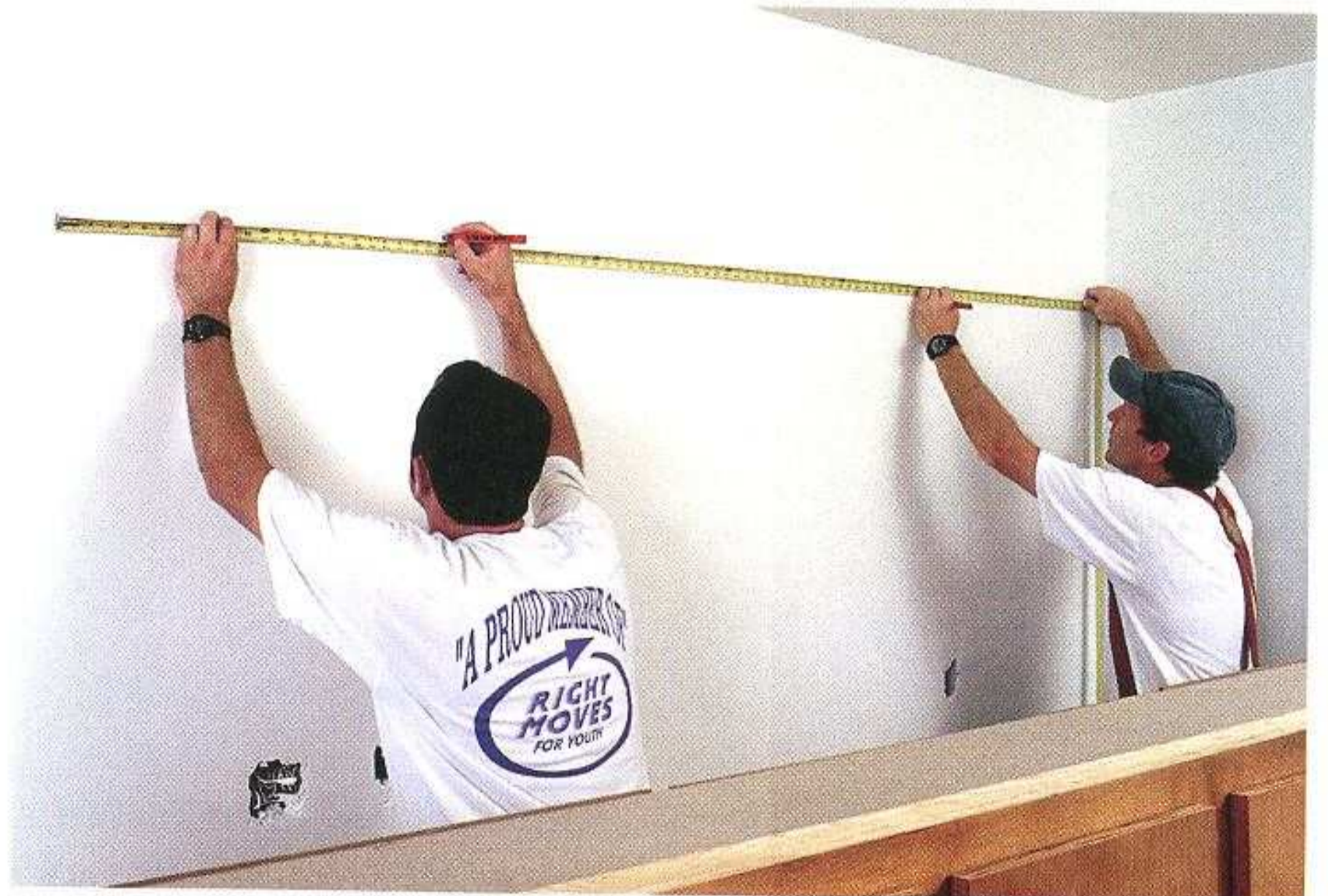
MEASURING AND MARKING. A steel tape measure is one of the most-used tools in a carpenter's kit.
