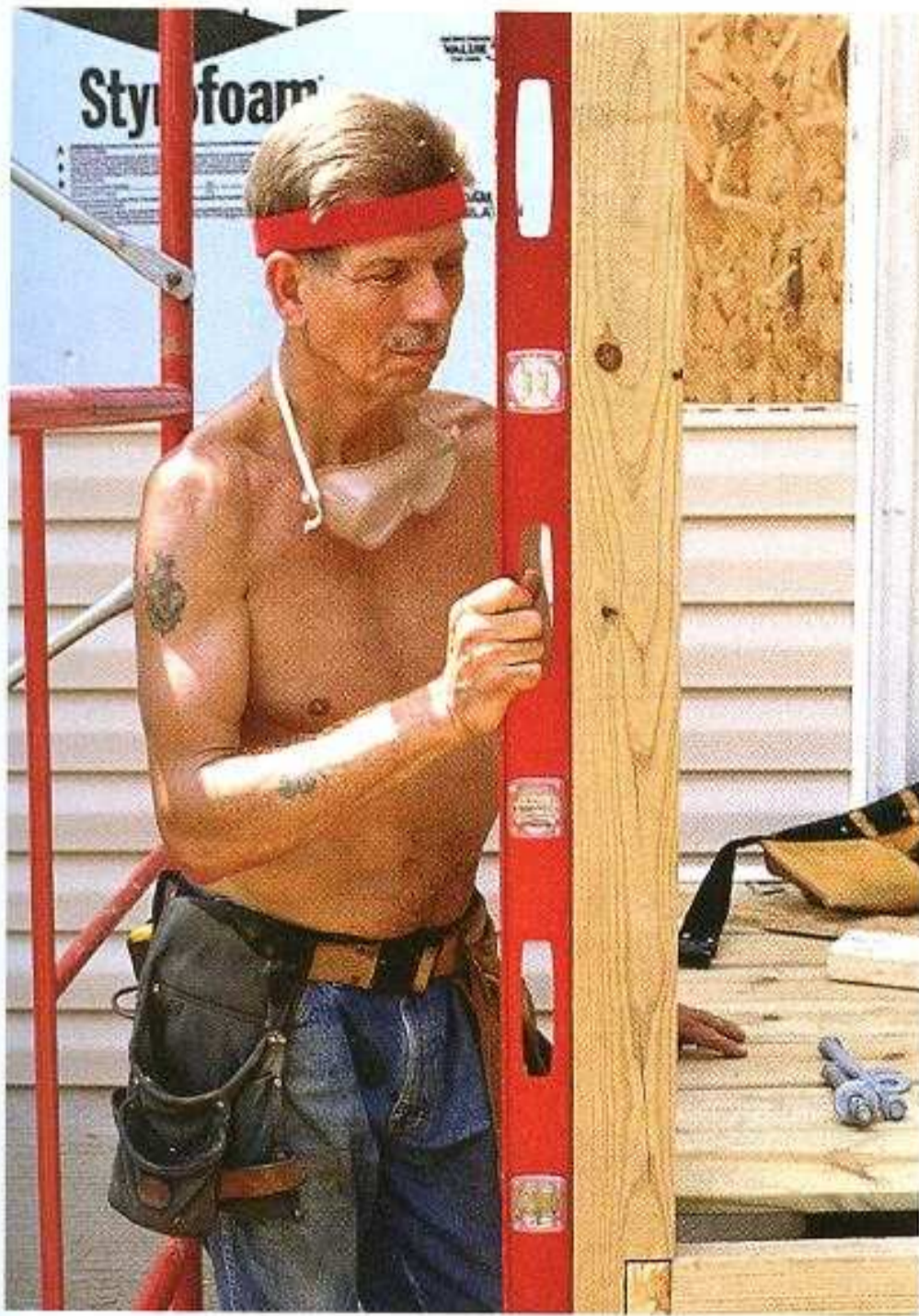
HORIZONTAL AND VERTICAL. Available in different lengths, levels can quickly test for plumb (vertical) and level (horizontal).
