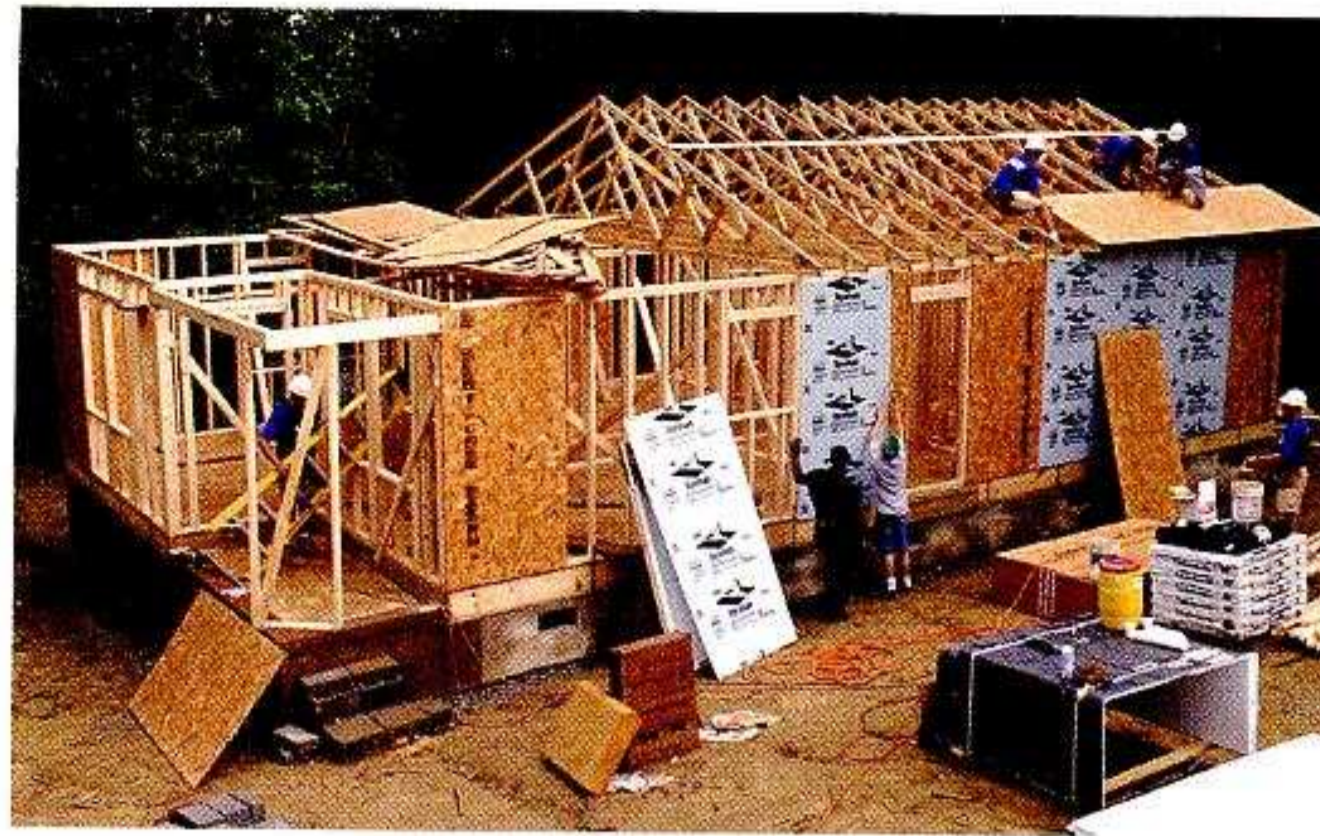
INSTALLING ROOF TRUSSES
