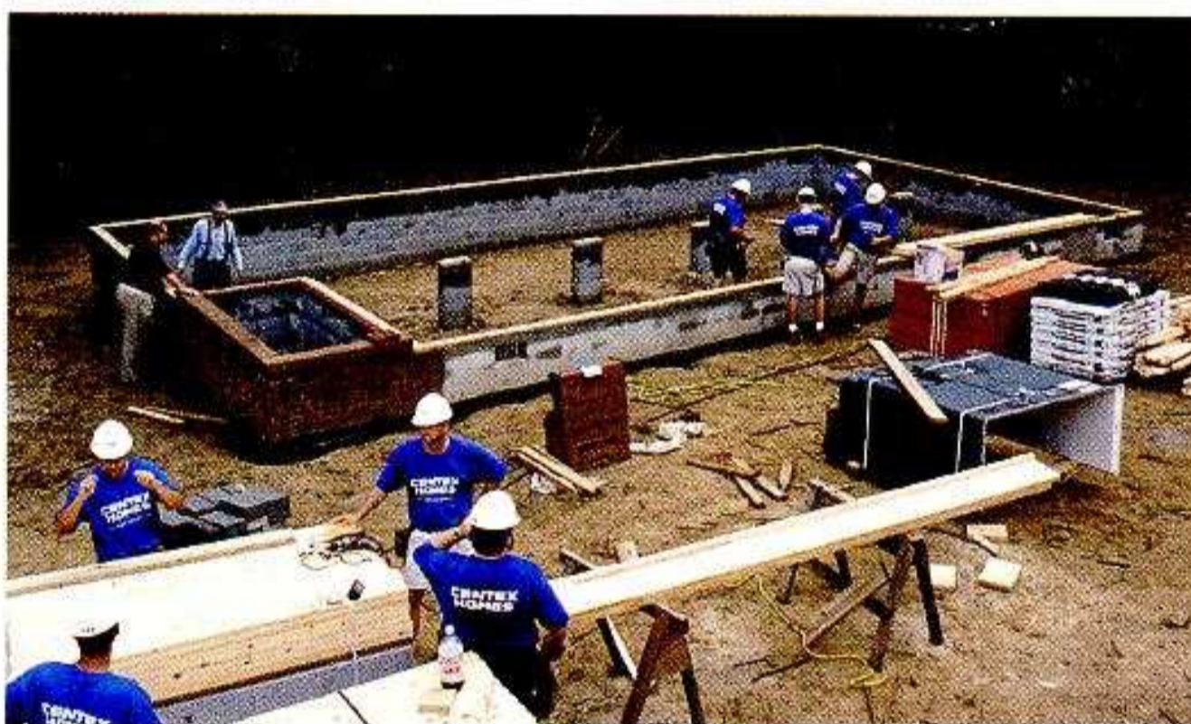
READYING THE FOUNDATION FOR FLOOR FRAMING
