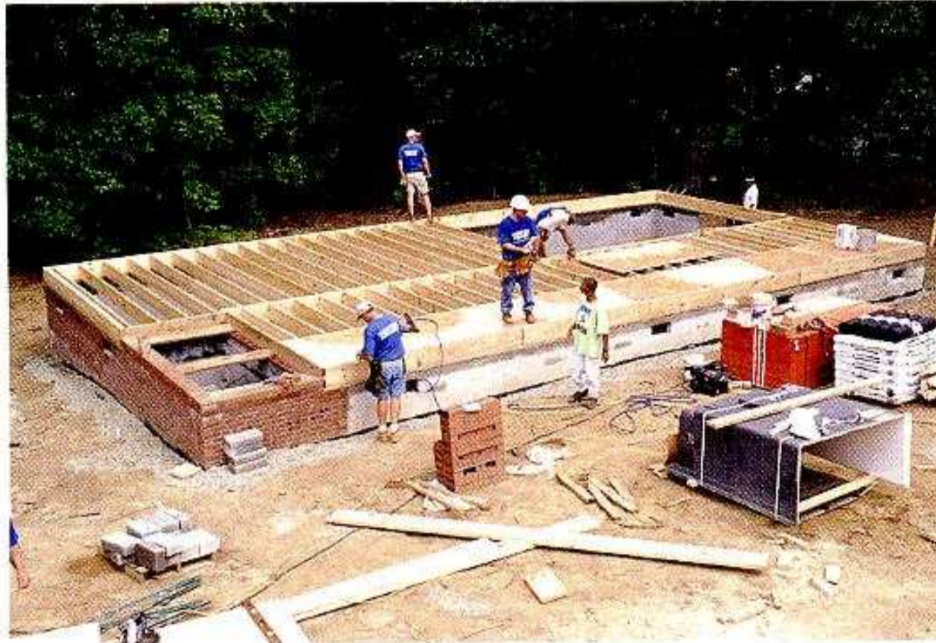
SHEATHING THE FLOOR
